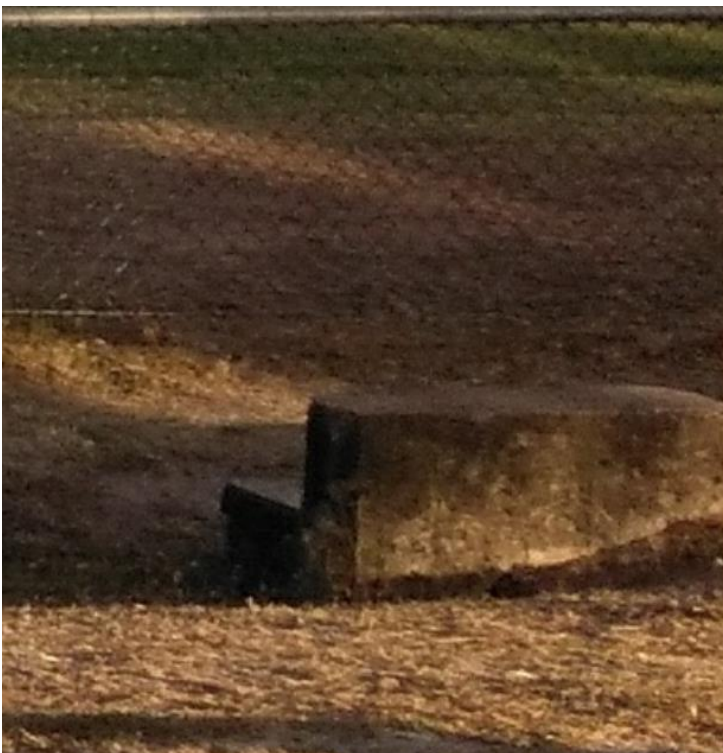
Figure 5 Concrete Inlet Structure on North- West Corner of Field
