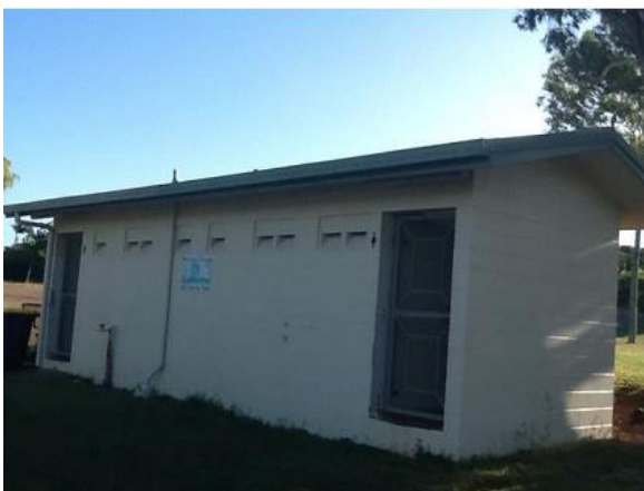
Figure 6 Existing Public Toilets
